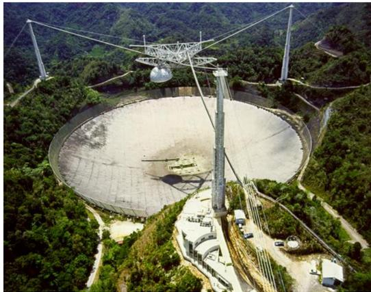
This is Arecibo observatory located in San Juan, Puerto Rico. Completed in 1963, Arecibo is part of the National Astronomy and Ionosphere Center (NAIC) funded by the NSF. The Observatory's 1,000 ft (305 m) radio telescope is the world's largest single-aperture telescope. The large dish reflects and focuses radio waves from the Universe.
