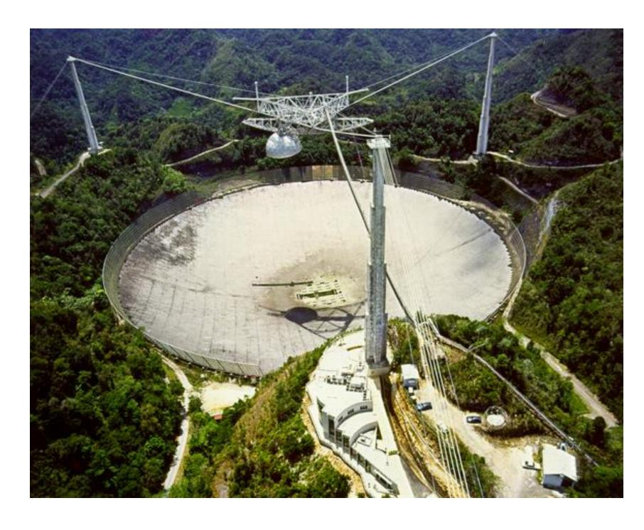
This is Arecibo observatory located in San Juan, Puerto Rico. Completed in 1963, Arecibo is part of the National Astronomy and Ionosphere Center (NAIC) funded by the NSF. The Observatory's 1,000 ft (305 m) radio telescope is the world's largest single-aperture telescope. The large dish reflects and focuses radio waves from the Universe.
